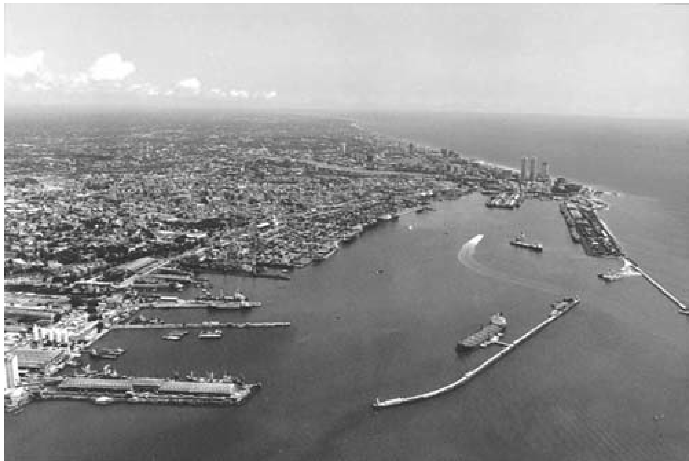
Port of Colombo, Sri Lanka, site of the "Colombo Plan" (1950). Japan assisted the port's expansion and improvement through yen loans and various other measures (Source: JICA)
