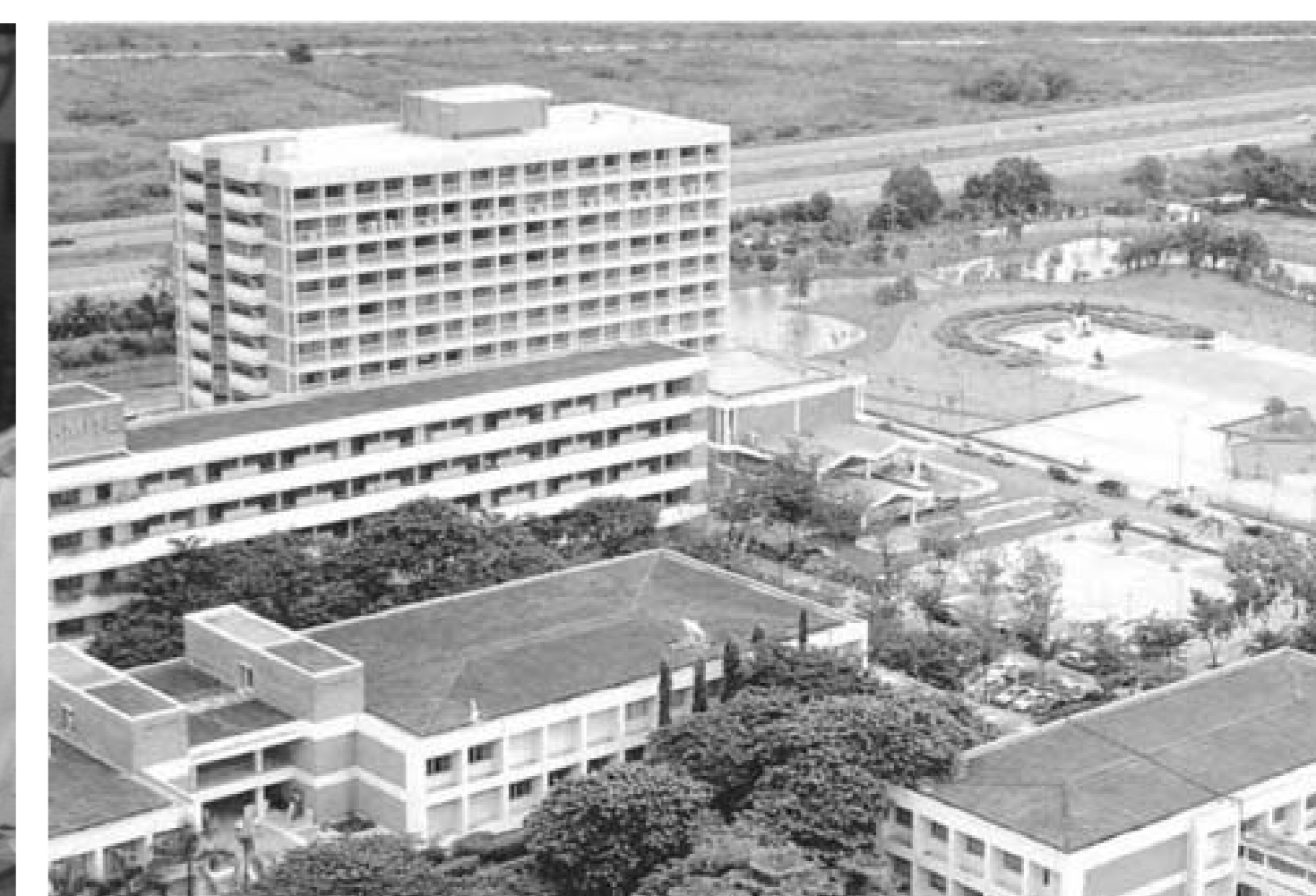
Nonthaburi Telecommunication Training Center, Thailand, 1960 (Source: JICA)
